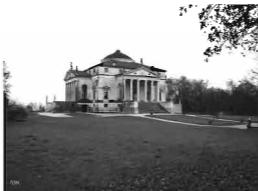
Fig. 7 The Rotonda and its surrounding landscape.
